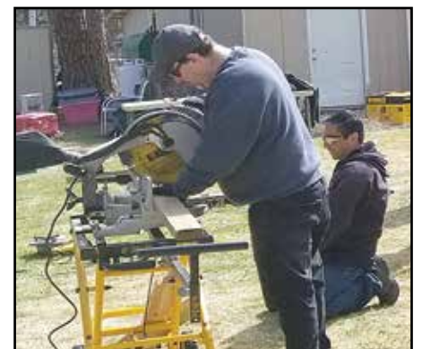
Cutting wood for the ramp railing.
