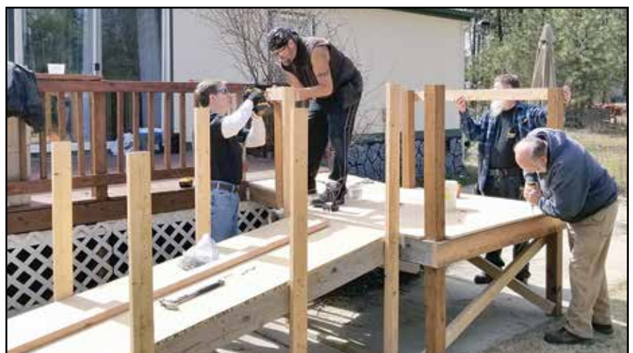
Volunteers building the ramp at Guyle's home.
