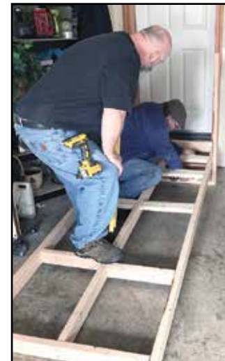
Left: Framing the Everett ramp.
