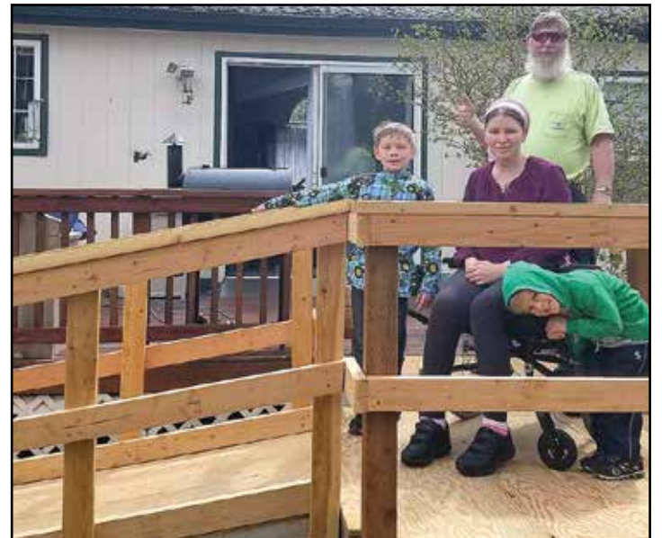
Above: Guyle Langlois (standing) poses on the finished ramp with daughter Ty and grandsons, Damian and Sava. With the ramp, Damian can bring Ty in and out of the house on his own.
