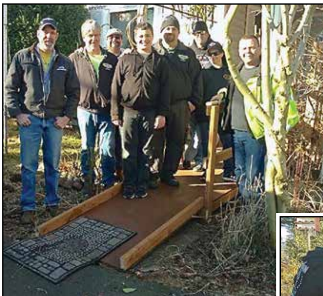
Above and right: Volunteers build a wheelchair ramp for a family in Everett.
