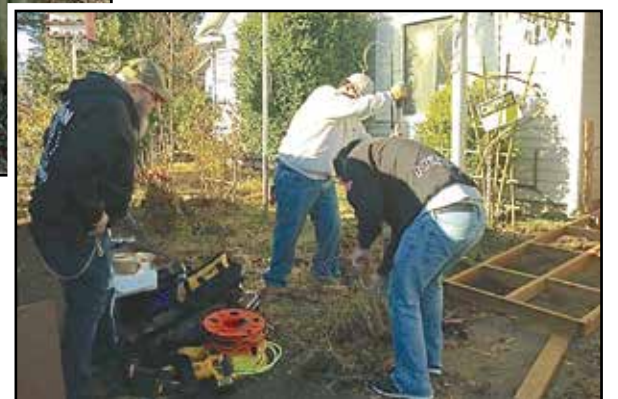
IAM 751 volunteers dig out the path for the wheelchair ramp frame for a family in Everett.
