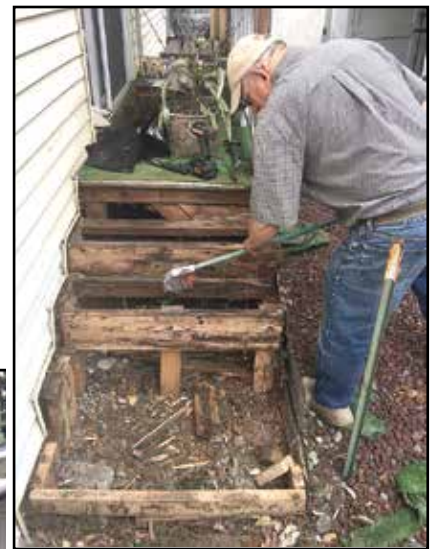
Above: Jim Hutchins tears out decaying steps and built new ones so a Federal Way resident can safely come and go from their home.
