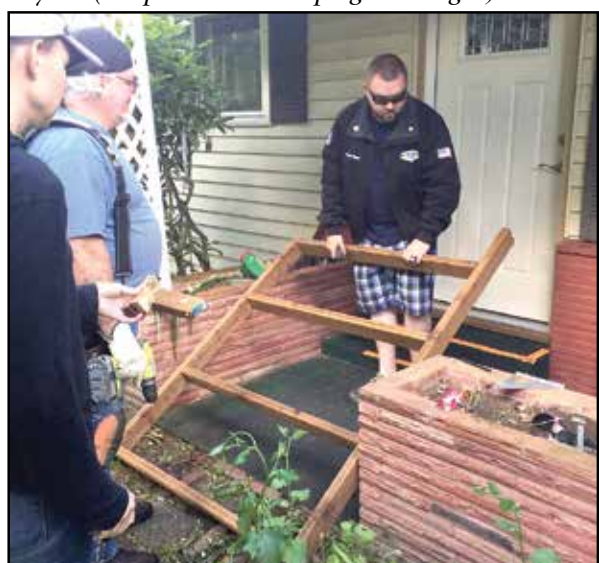
David Wyatt installs a hand rail.
