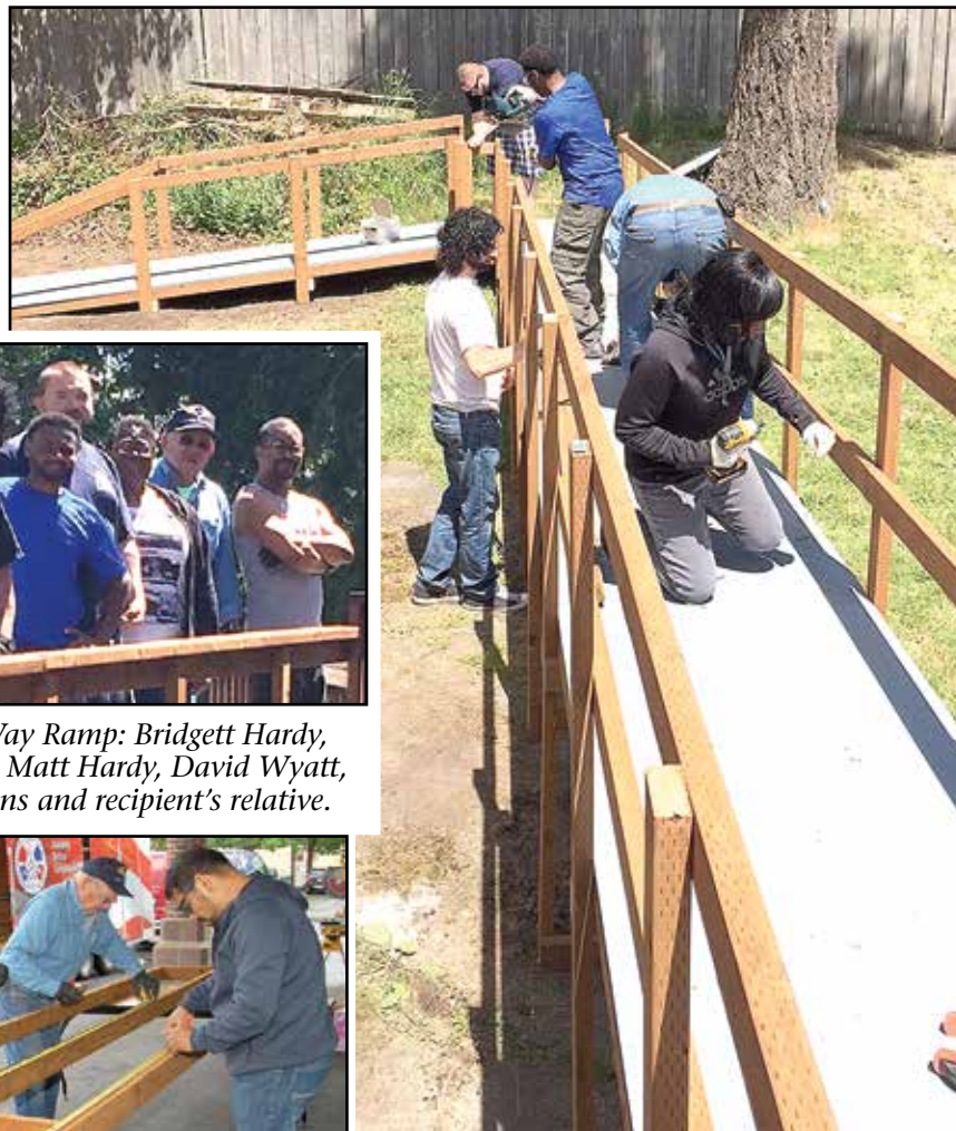
The Federal Way ramp was long to ensure the grade wasn't too steep for the resident.
