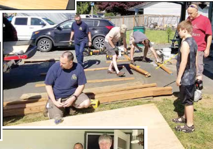
Above: Volunteers cut the wood for the Marysville ramp. Left: Volunteers stand on the completed ramp along with the resident. L to R: Derek Gottschalk, Adrian Camez, Steve Morrison, Seth Hill, Jason Redrup, Ed Page, Mike Hill and Paul Richards. (Also helped but not pictured Carl LaPlante).
