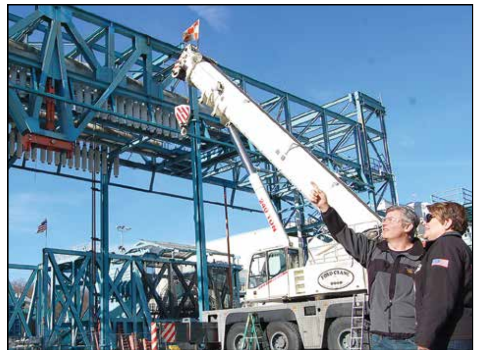
Steward George Stefanini and Business Rep Grace Holland look at the approximately 2,000 hours of demolition work our members will perform taking out the infrastructure, thanks to the union speaking up and stopping a contractor from performing what has traditionally been our work.
