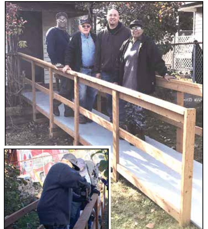
Volunteers who traveled to Bremerton to build a recent ramp included: Princie Stewart, Jason Chan, Jim Hutchins, Jack Young and Ed Lutgen.
