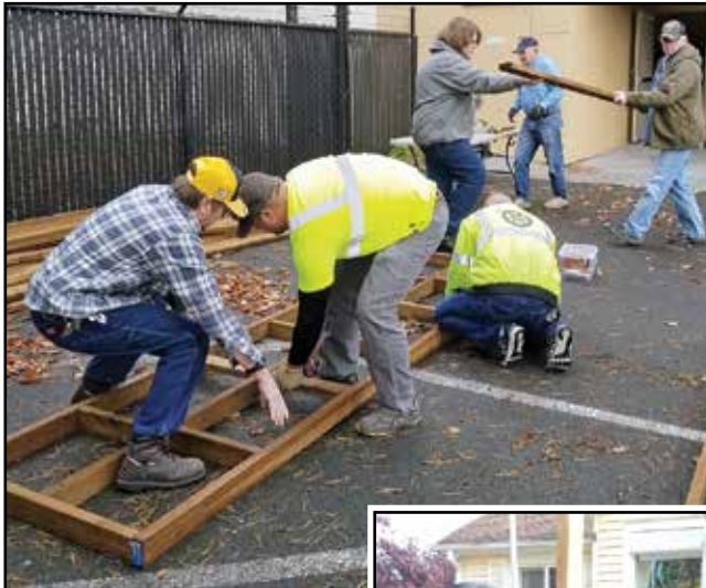
Above: Volunteers pre-build parts of the wheelchair ramp to make the actual build and installation go quicker. Right: The next generation of Machinists' volunteers helped with the ramp project.
